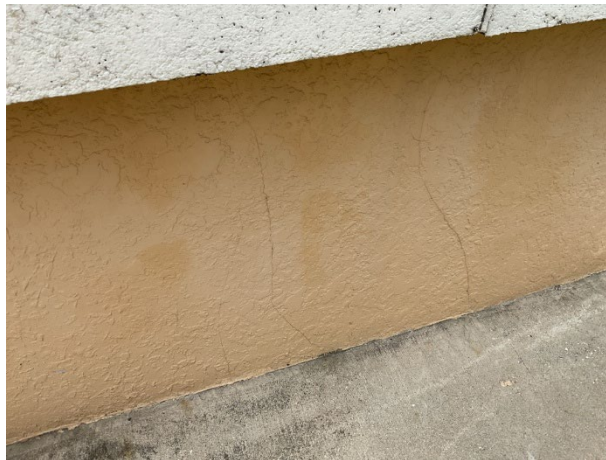
Stucco cracks
