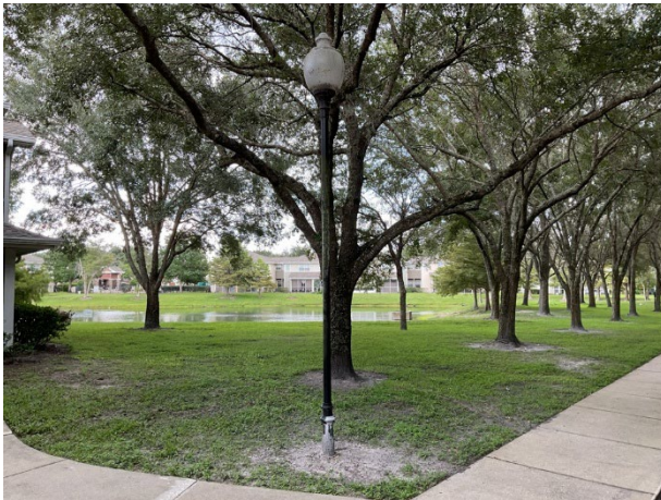
Light pole and fixture
