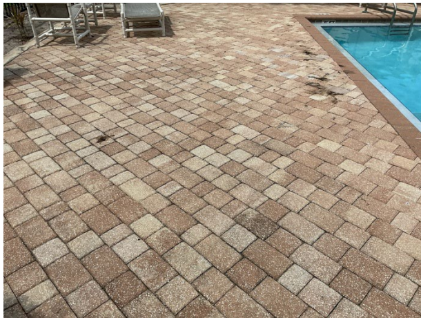
Paver pool deck overview
