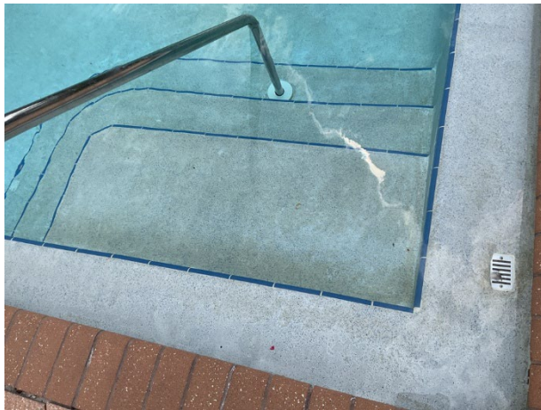
Pool plaster finish with tile perimeter
