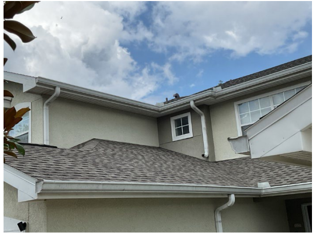
Roof overview at units
