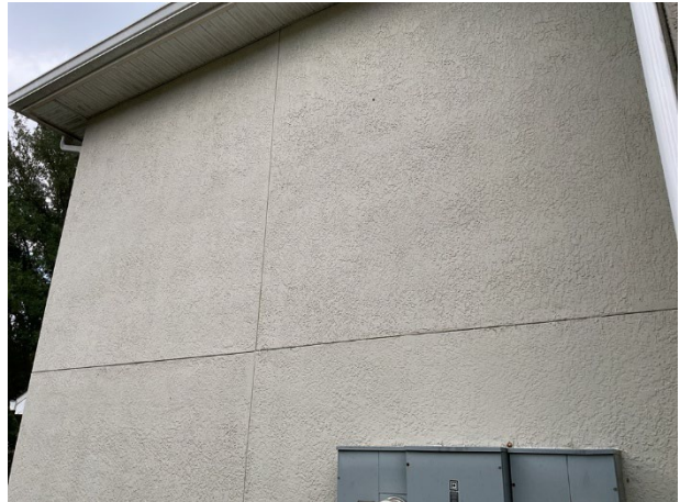
Stucco wall finishes
