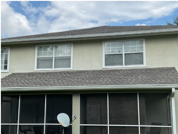
Roof overview at units
