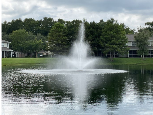
Pond fountain aerator
