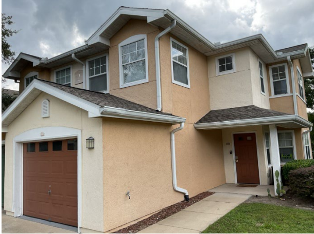
Aluminum gutters and downspouts
