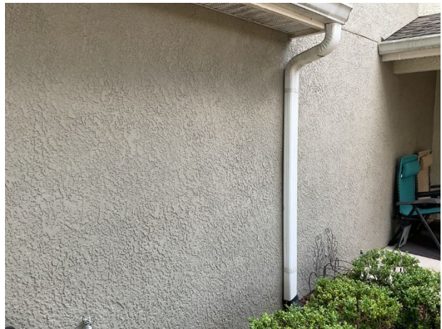
Stucco wall finishes
