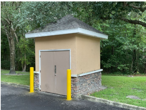
Storage building overview
