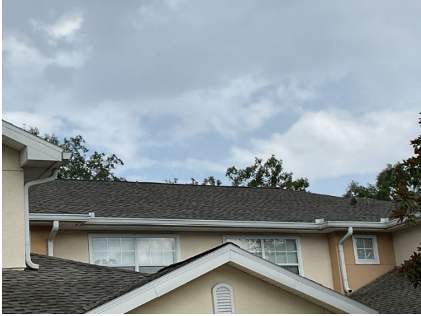
Roof overview at units
