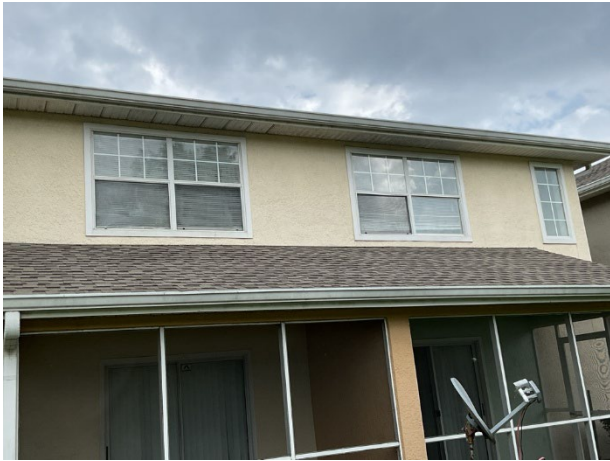
Roof overview at units
