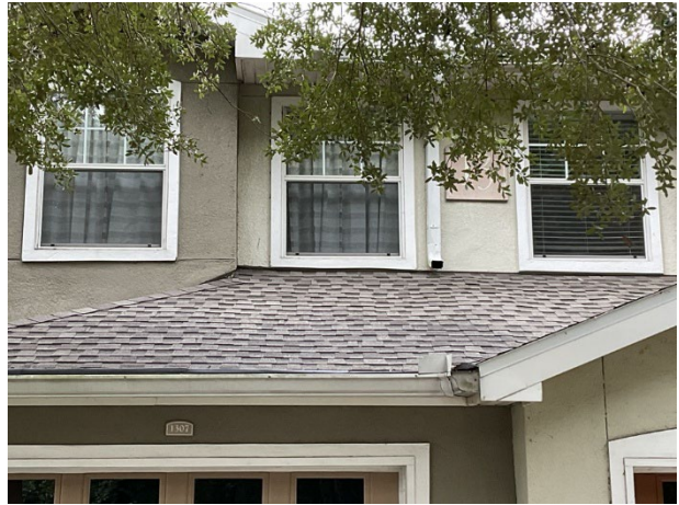
Roof overview at units
