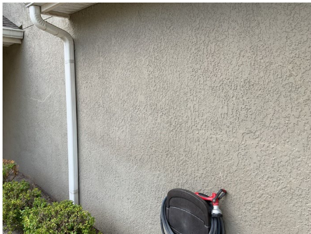
Stucco wall finishes
