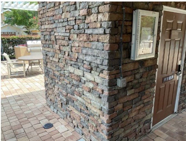
Masonry walls overview at pool house
