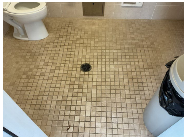
Pool house restroom tile flooring
