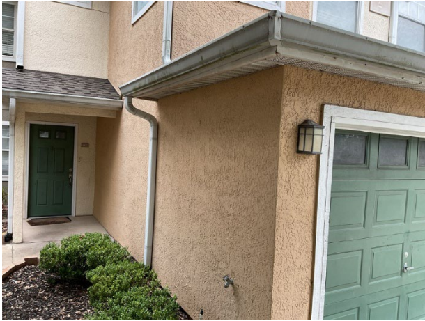
Aluminum gutters and downspouts
