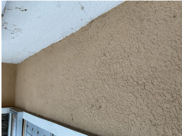
Stucco wall finishes at mailbox station
