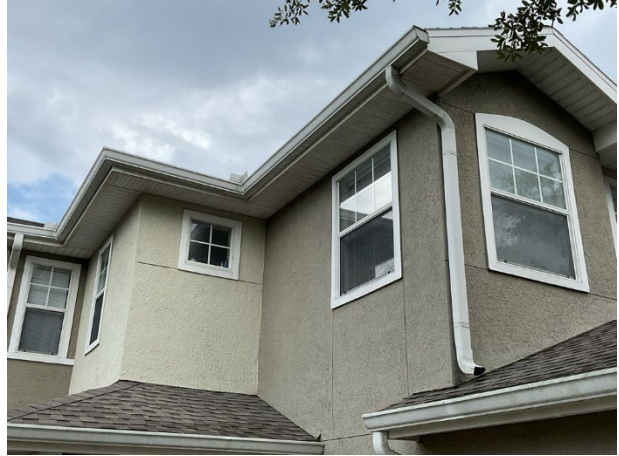
Aluminum gutters and downspouts
