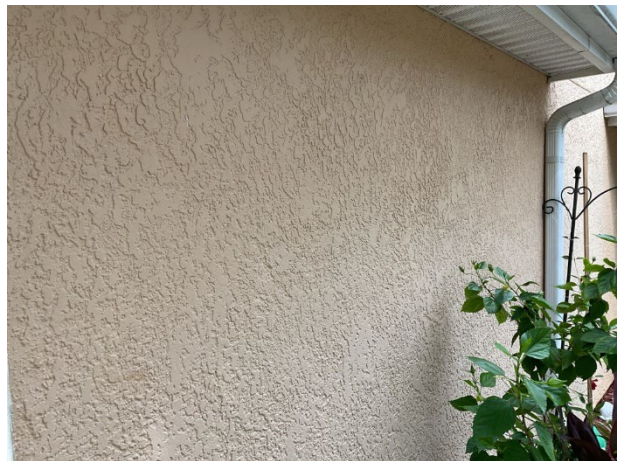
Stucco wall finishes
