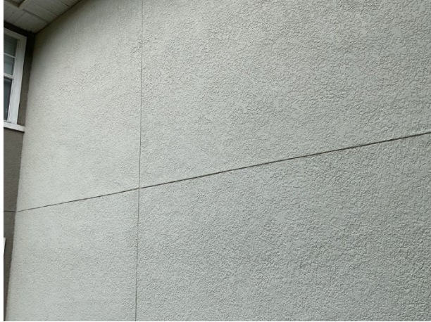
Stucco wall finishes
