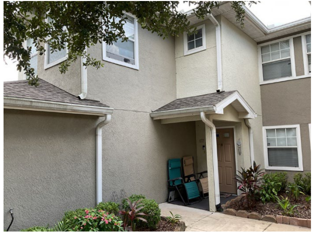
Aluminum gutters and downspouts
