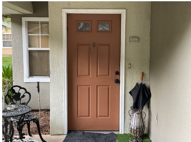
Unit entrance door
