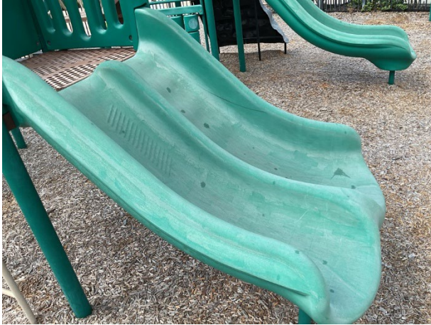
Equipment finish deterioration
