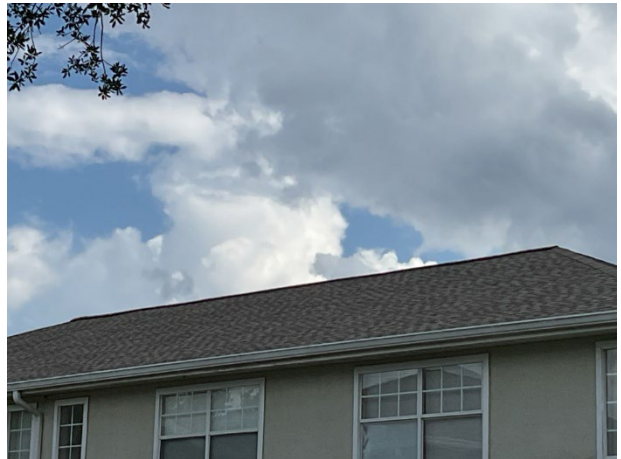
Roof overview at units
