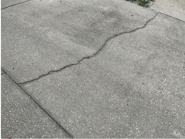
Driveway cracks
