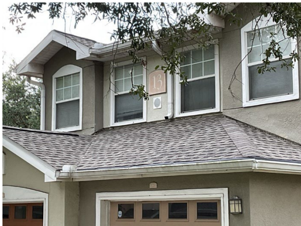
Roof overview at units
