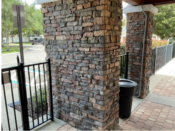
Masonry pillars overview at pool house
