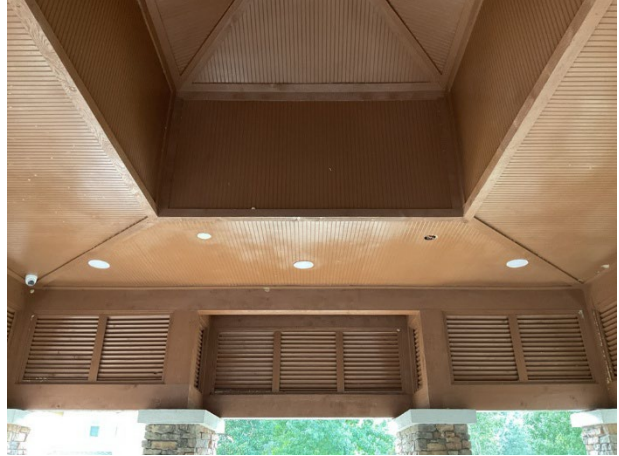
Pool house wood ceiling
