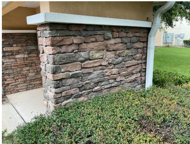
Masonry walls overview at mailbox station
