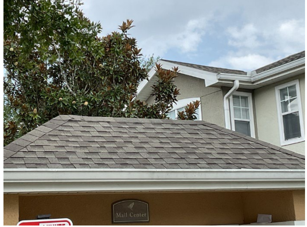
Mailbox station roof
