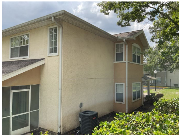
Aluminum gutters and downspouts
