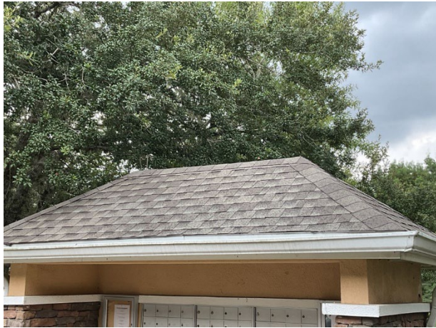
Mailbox station roof
