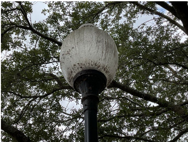
Light pole and fixture
