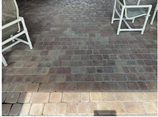
Paver pool deck overview
