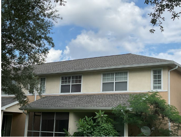
Roof overview at units
