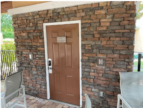
Masonry walls overview at pool house
