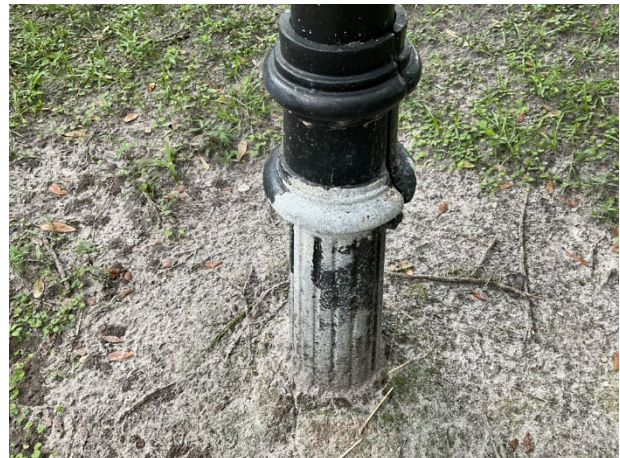
Finish deterioration
