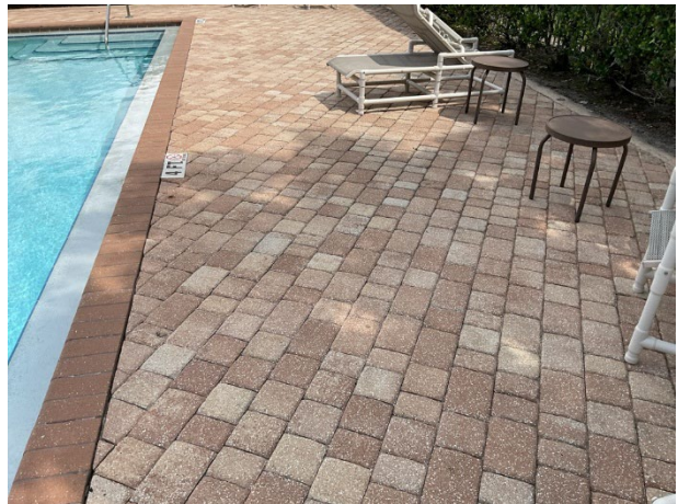
Paver pool deck overview
