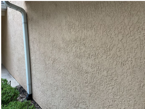
Stucco wall finishes
