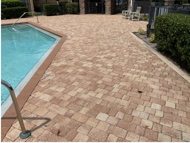
Paver pool deck overview
