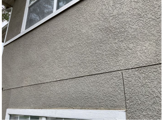
Stucco wall finishes
