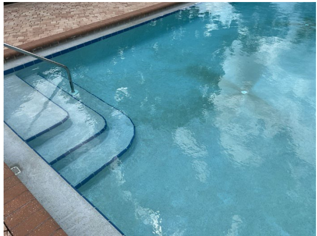
Pool plaster finish with tile perimeter
