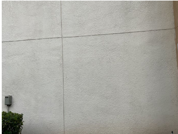
Stucco wall finishes
